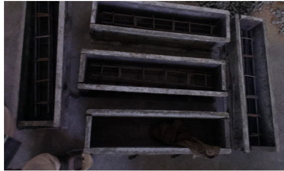
Figure 3 Mould preparation
