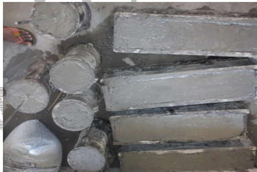
Figure 2 Casting of RCC beams
